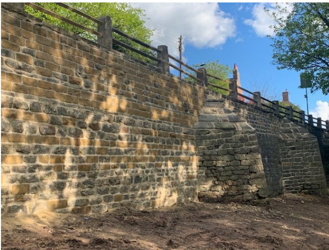
Mill Bank walls repaired
